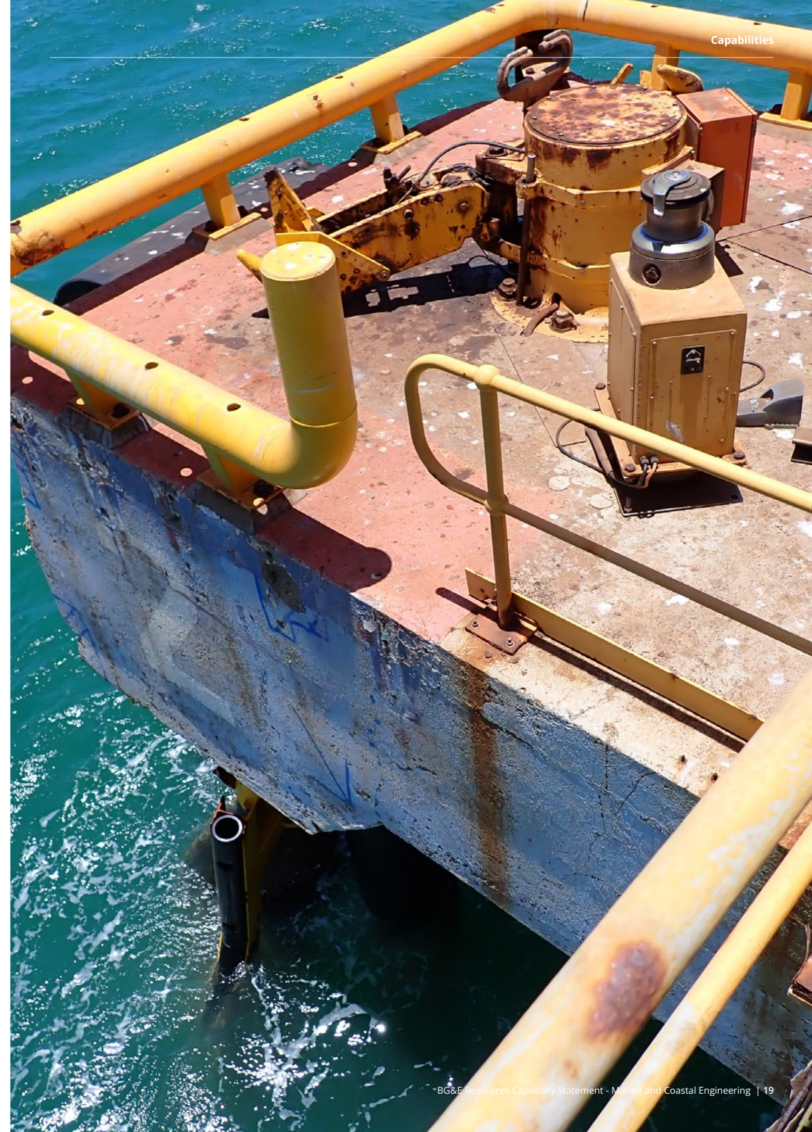
Image: Dampier Jetty Structural Inspection.
