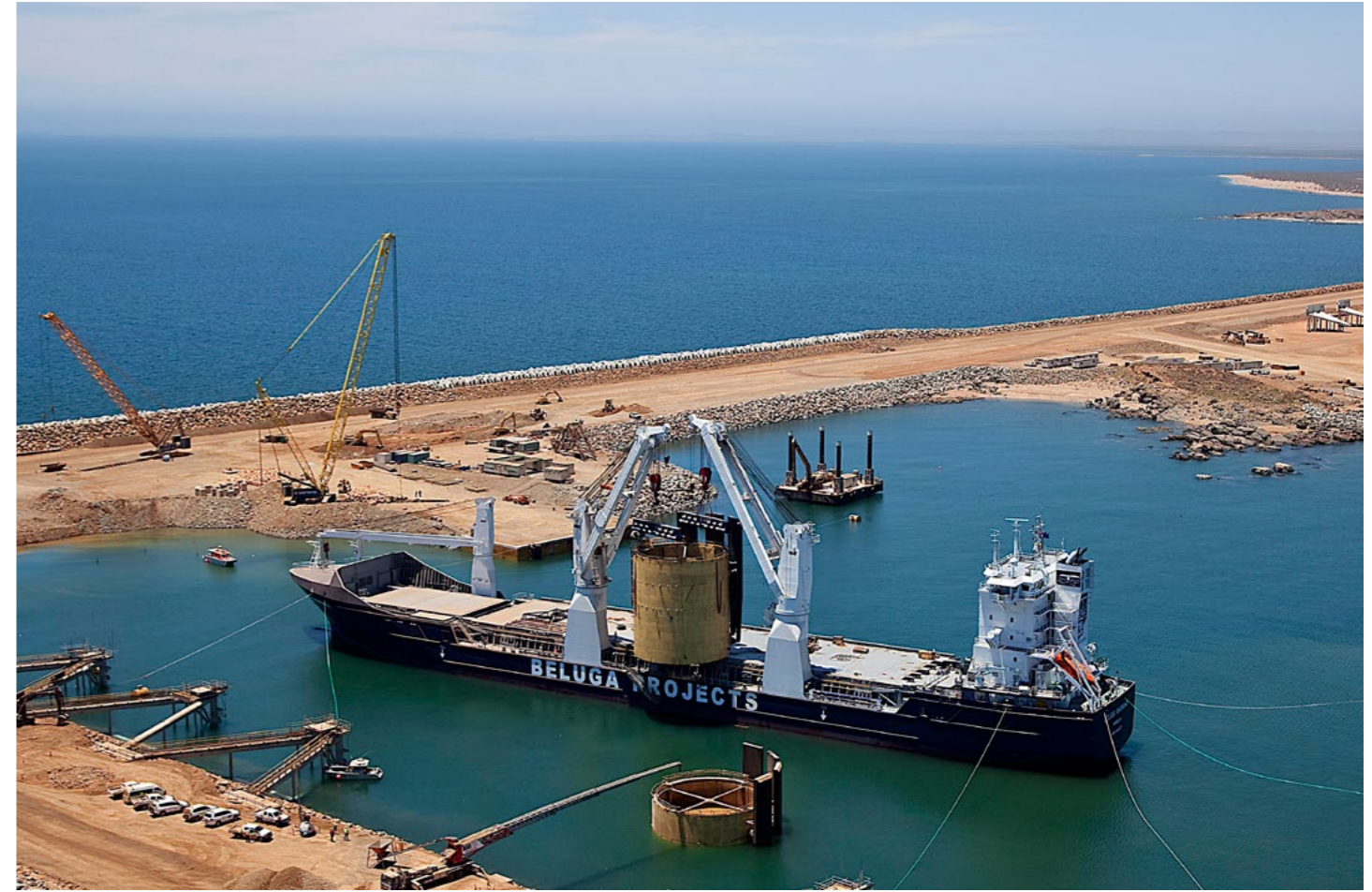
Image: Cape Preston Lift - Cape Preston, WA.
