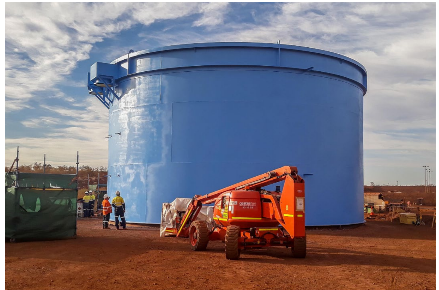
Brockman 4 Mine, Pilbara WA.
