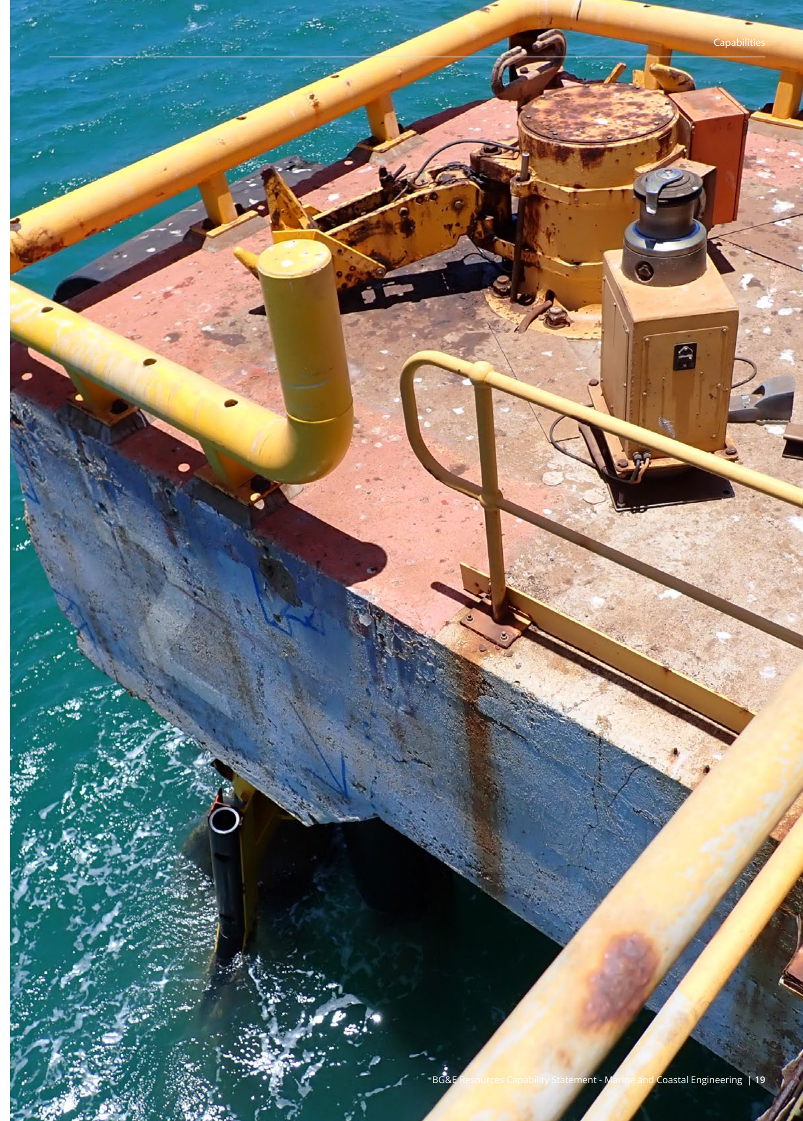
Image: Dampier Jetty Structural Inspection.
