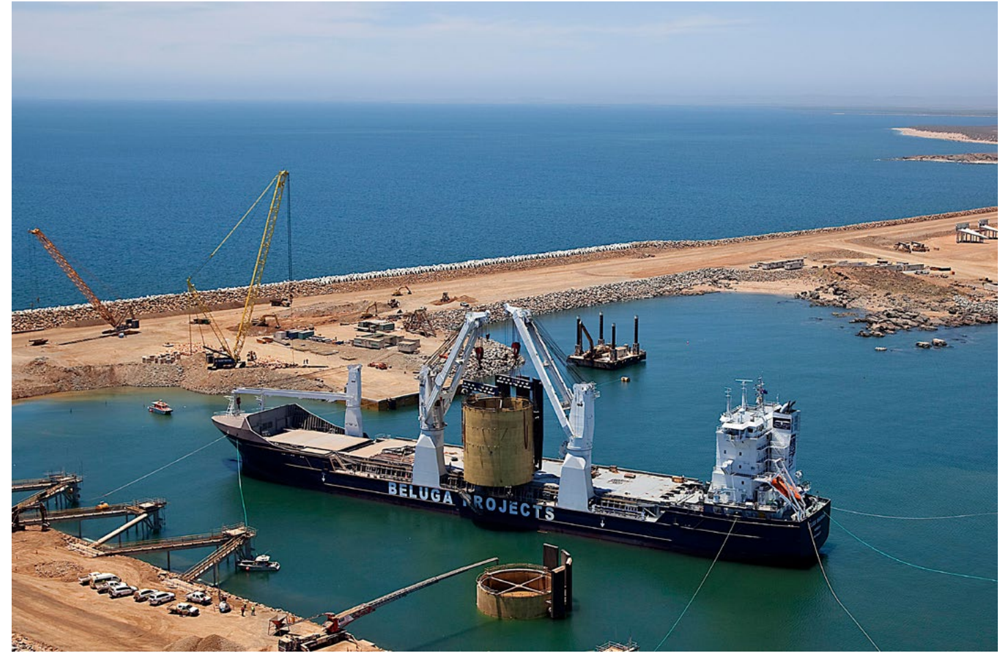
Image: Cape Preston Lift - Cape Preston, WA.
