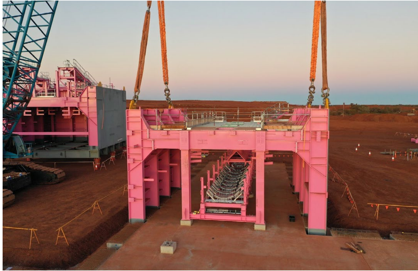
Image: Structural Integrity & Asset Inspection - Lake MacLeod, WA.
