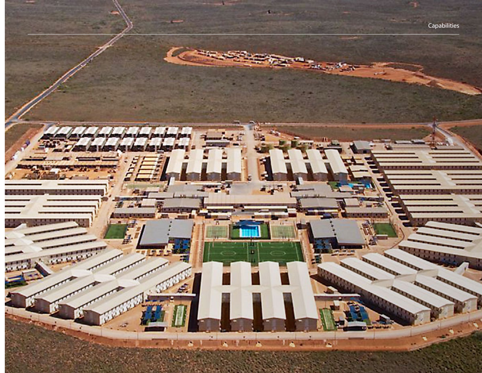
Image: Decmil Gorgon LNG Barrow Island Accomodation – Barrow Island, WA.
